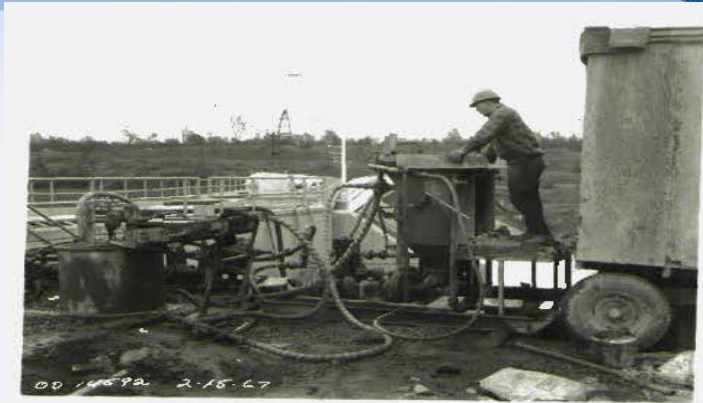
Photo No. 31. Grouting equipment. High speed, double drum grout mixer is on right; agitator is on left. Grout pump is behind agitator. View towards left abutment. Neg. No. OD 14592 2-15-67
